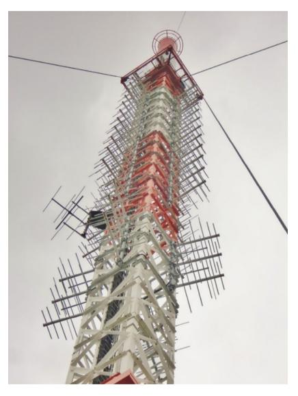
*in the picture: Low wind load FM LogPer antennas at the "Wittenberg" station*
